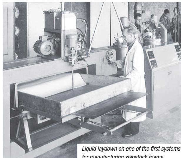
*Liquid laydown on one of the first systems for manufacturing slabstock foams*
